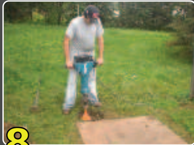
Backfill & Tamping
