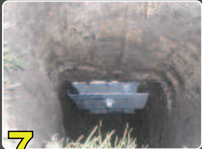
Anchor Torqued & Seated
